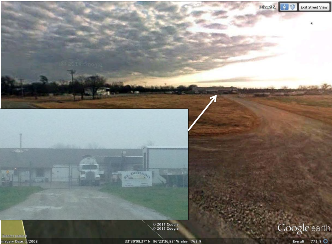
El Dorado Chemical Plant (Whitewright, TX)
