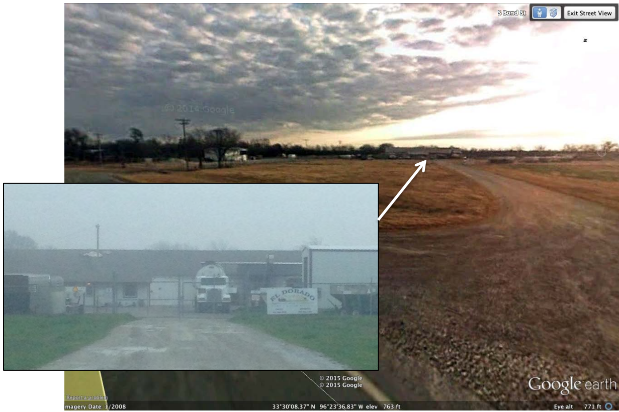
El Dorado Chemical Plant (Whitewright, TX)
